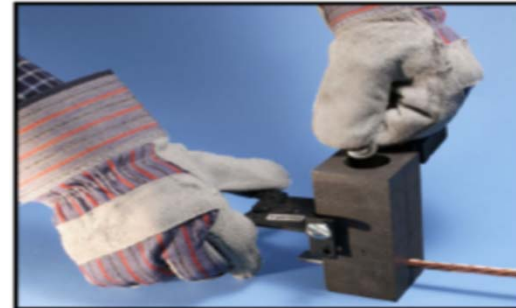
Removing Oxidation from the grounding Busbar
