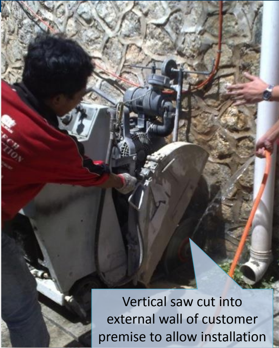
Installation of raceways at customer premises
